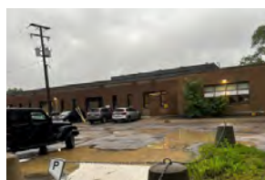
Pinewood Elementary Before
