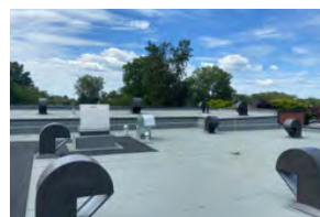
Mountainview Elementary After
